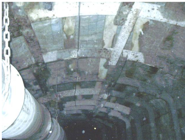
Sets scribed with voidcrete installed
