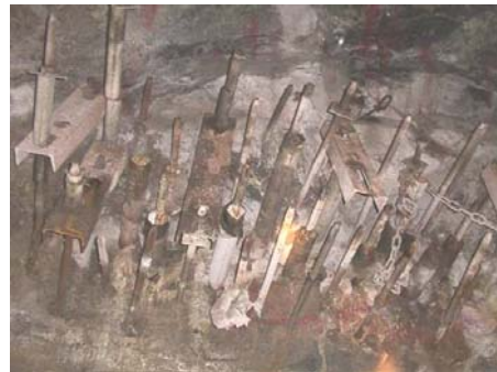
Spiling casing pipes
